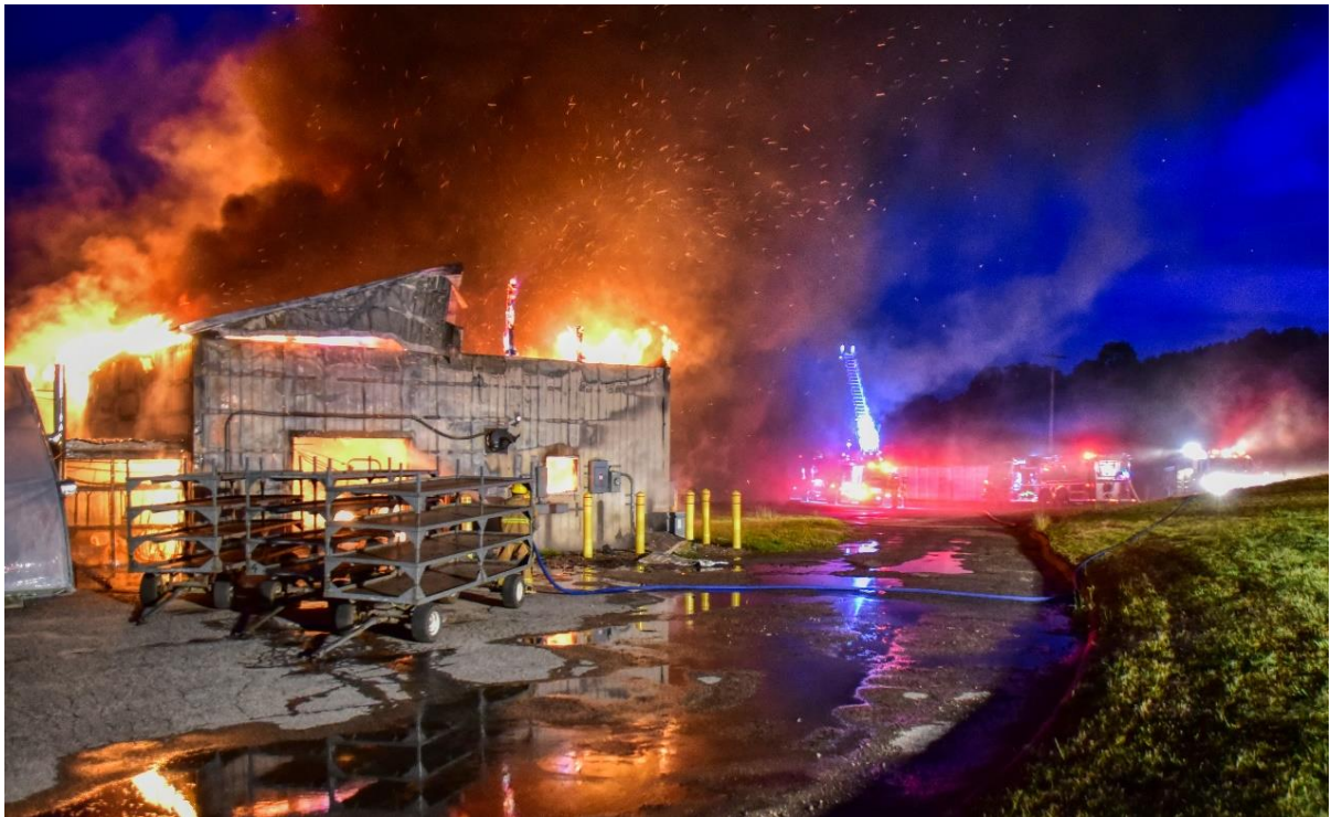
Franklin, Ct Commercial Building fire 06-24-24 Photo by Robert Ladd
