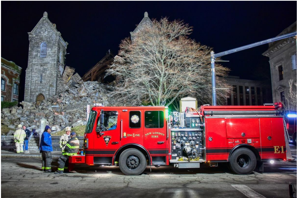
New London, Ct Church collapse Photo by Robert Ladd
