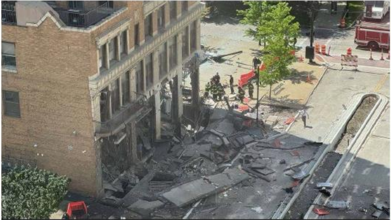
Aftermath of the explosion. Photo by John White
