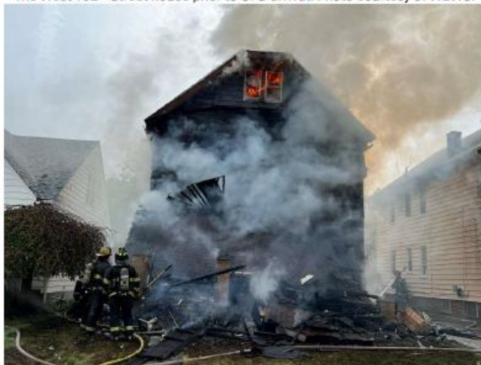
The house after the collapse. Photo courtesy of the CFD.
